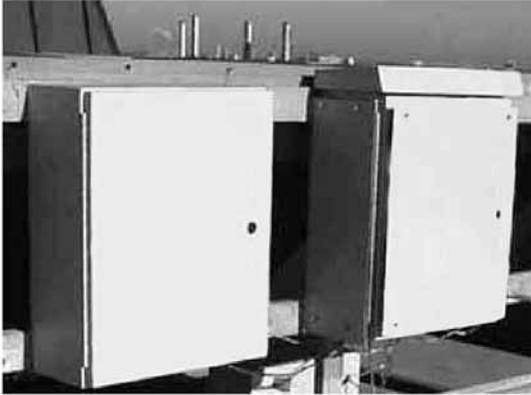
Hoffman’s research on the effects of solar radiation on enclosures has shown the positive benefits of utilizing shielding to decrease temperature rise. Shielding has been found to be an effective, low-cost method of reducing solar heat gain in outdoor electrical/electronic applications.
